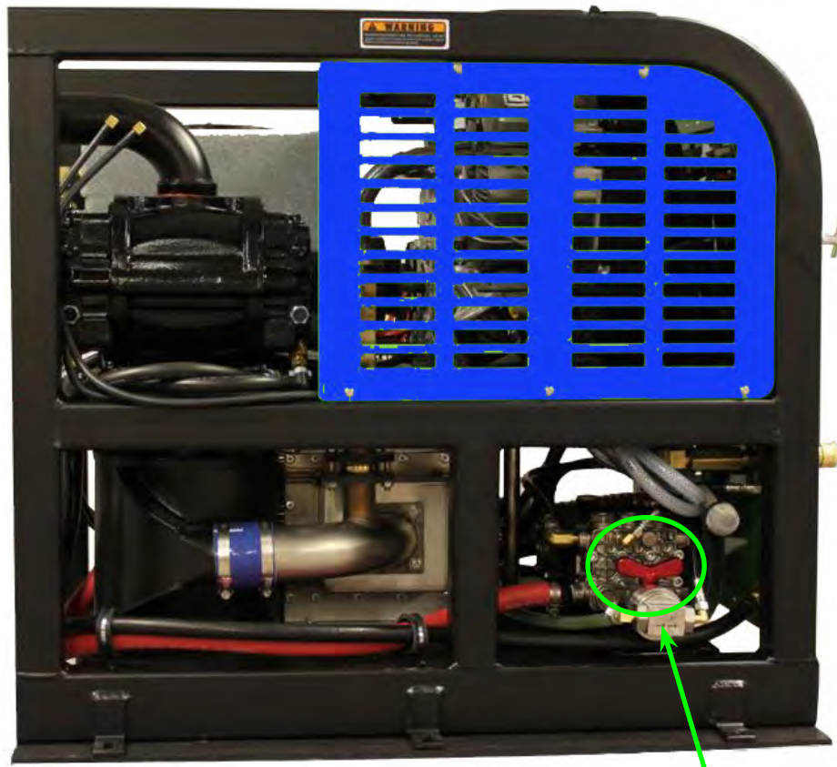
Chemical Pump Shutoff Valve
